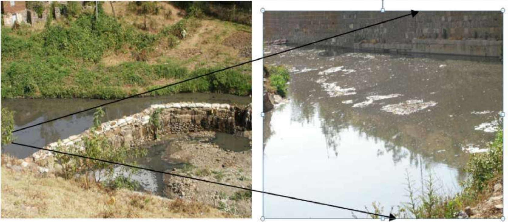
Figure 8. Diversion structure from Kera tributary(December 9,2010)
